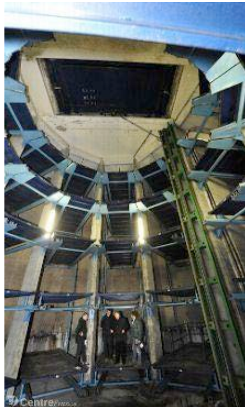
Parking silo de Chamalières
